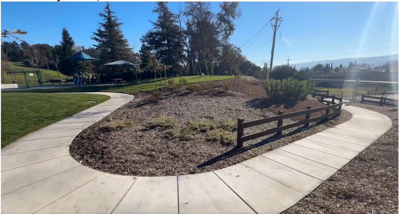
Photo 4. Project area, after construction
