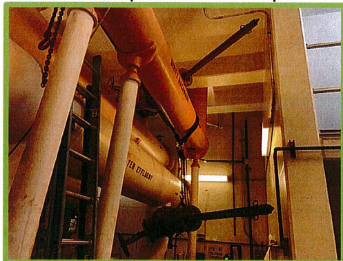
Installation of Line Stops
