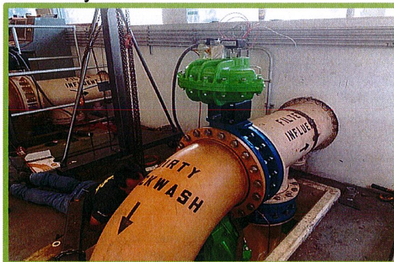
Installation of new Pneumatic Valves
