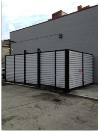
Figure 19 - Roanoke, VA Enclosure
