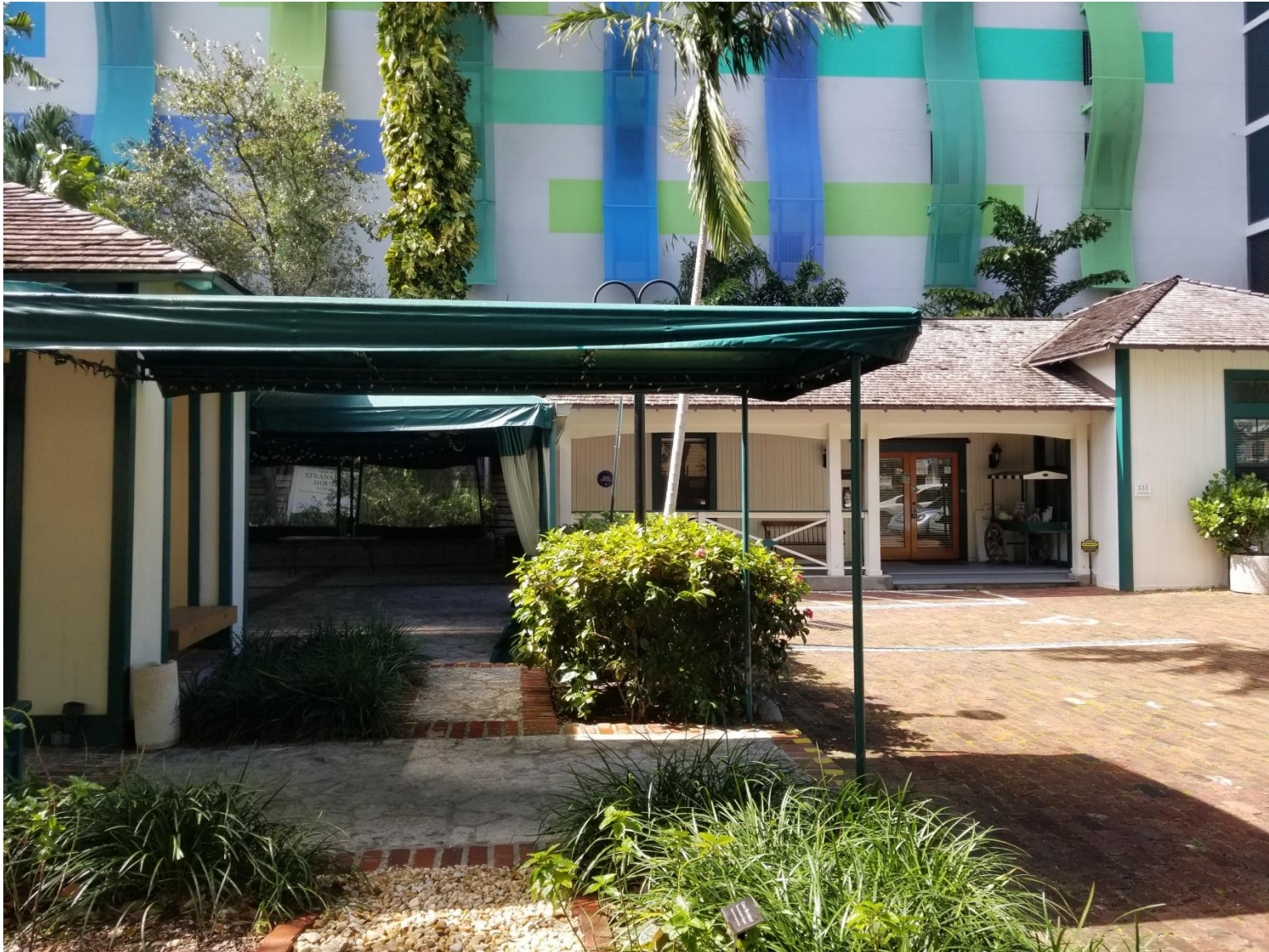
STRANAHAN HOUSE COURTYARD AND CANOPY – FACING WEST
