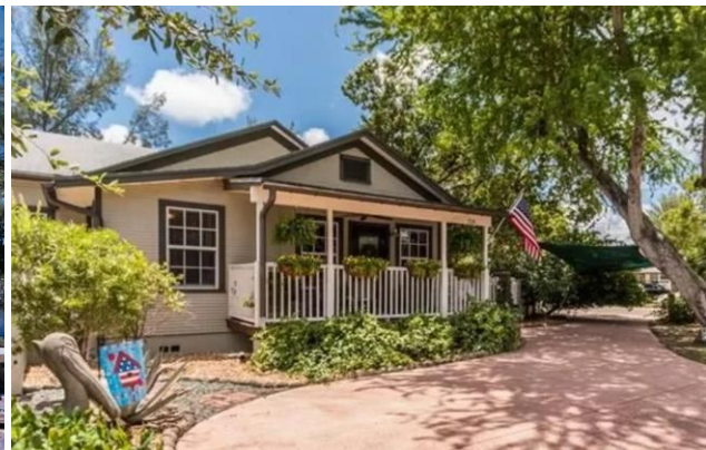
Current photo of front (north) elevation
