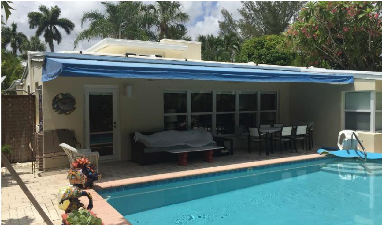
Current Photo of Rear Elevation
