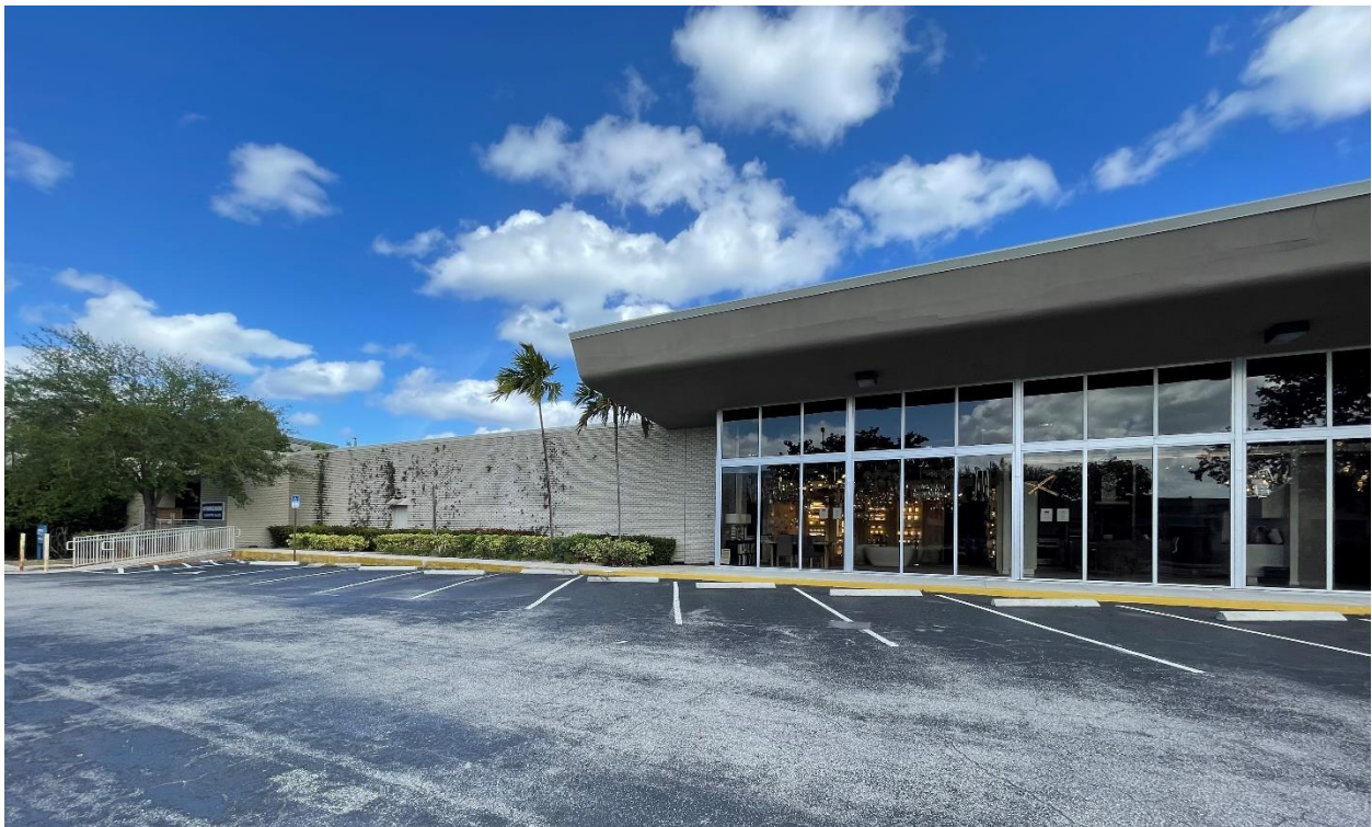
Front Elevation Looking Northeast
