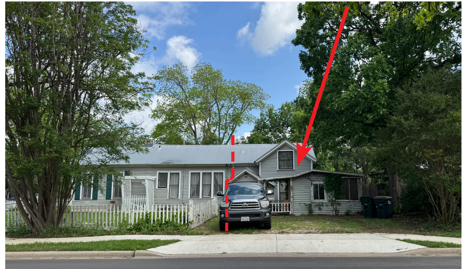
SOUTH FACADE FACING 15 ST
