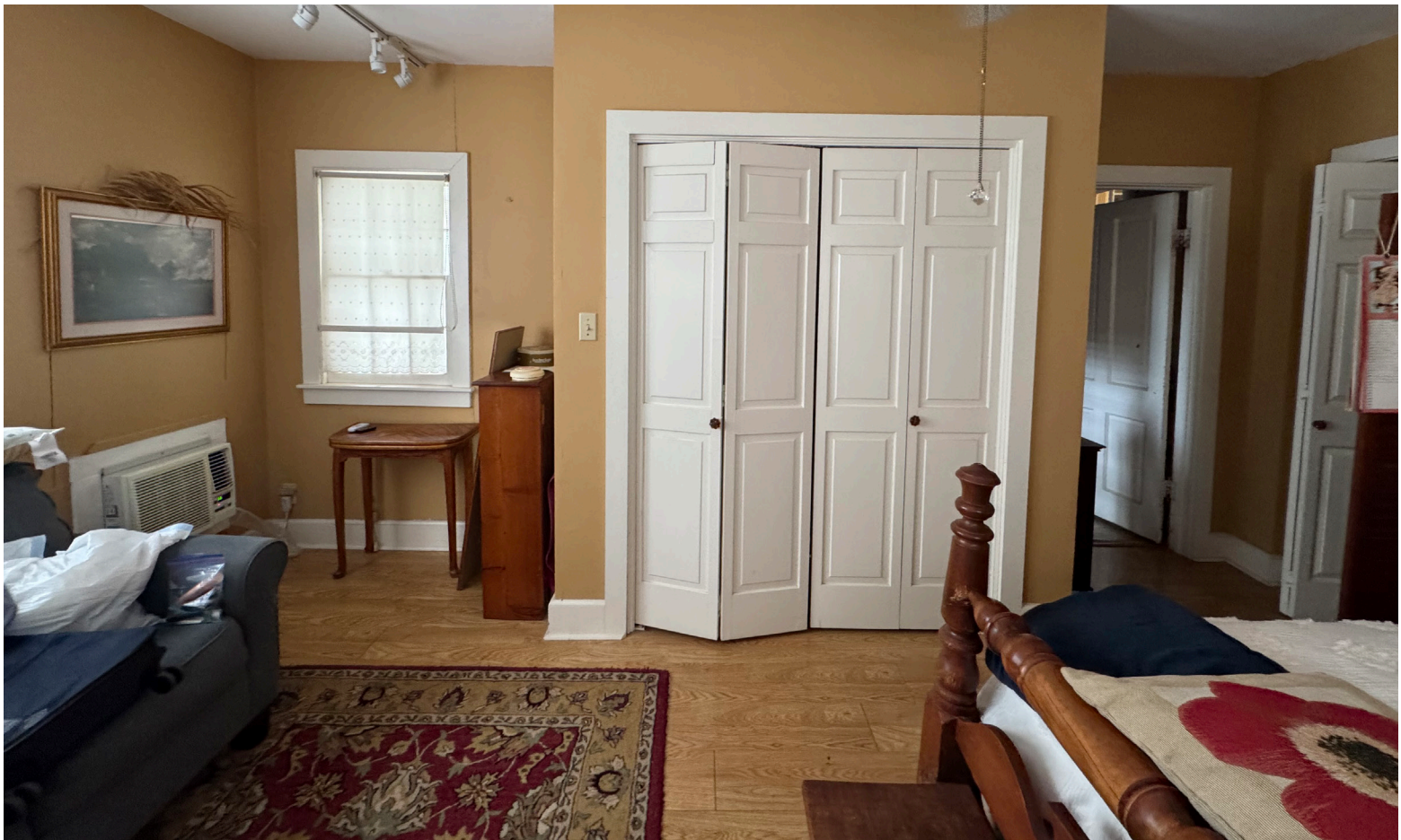
1970S BEDROOM W/ LINOLEUM FLOOR TO BE REMOVED
