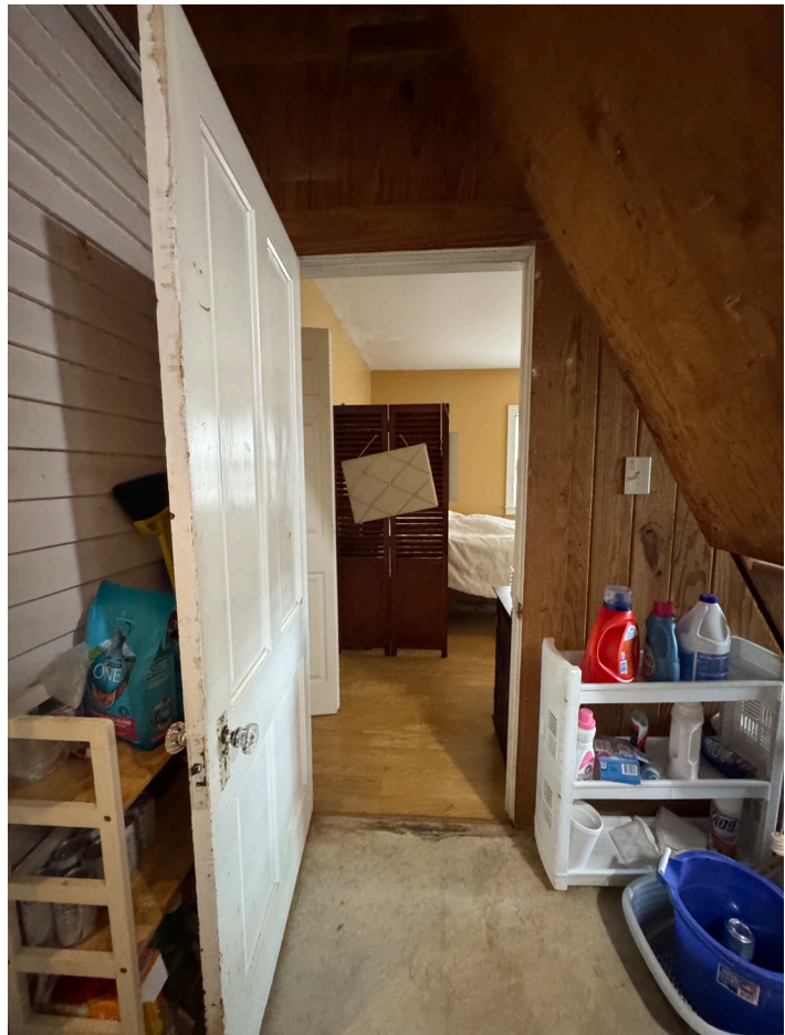
1970S HALLWAY AND STAIRS: TO BE REMOVED
