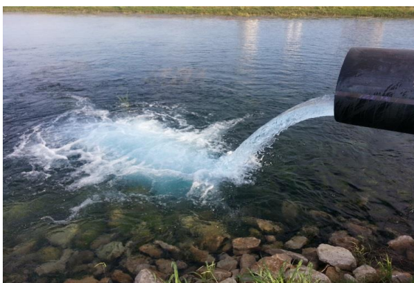
Figure C.6 RO permeate (Photo credit: City of Wichita Falls)
