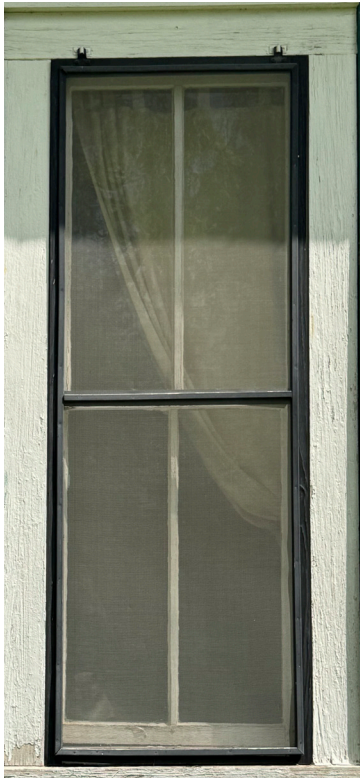
EXISTING WINDOWS TO BE REPLACED ALL SHUTTERS + SCREENS TO BE REMOVED
