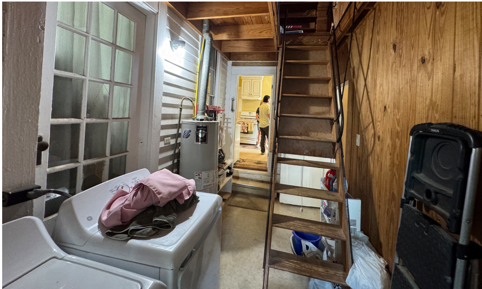
1970S HALLWAY: TO BE REMOVED
