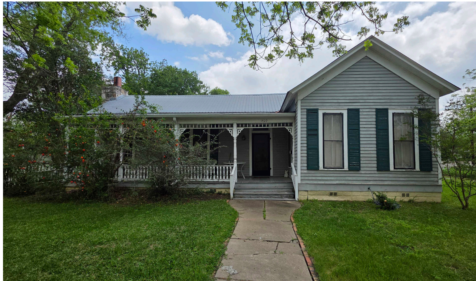
WEST FACADE FACING OLIVE ST
