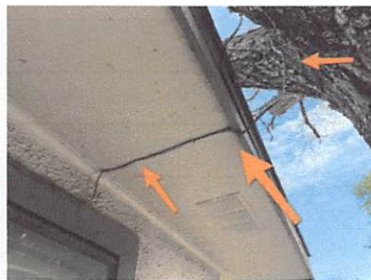
Exposed and unprotected wiring
