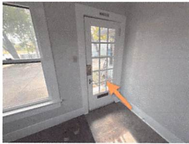
No tempered glass etching observed at left side exterior door
