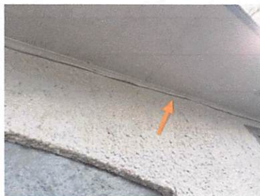
Exposed and unprotected wiring
