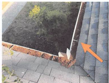
Clear debris from gutters
