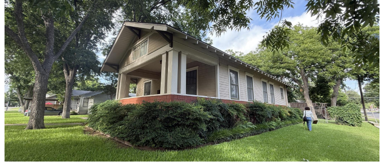
VIEW OF NORTHEAST CORNER OF E. 10TH & ELM STREET
