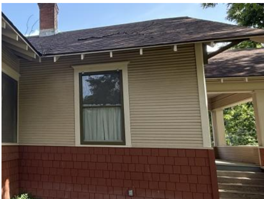
VIEW OF EXISTING SIDING INCLUDING 3" CLAPBOARD, AND SHAKER SHINGLE SKIRTING TO MATCH NEW CONSTRUCTION. 4" TRIM AROUND CORNERS AND WINDOWS WITH CRAFTSMAN WINDOW CAP MOULDING
