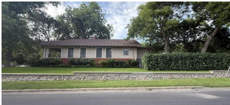
VIEW OF NORTH FACADE OF HOUSE FROM E. 10TH ST.
