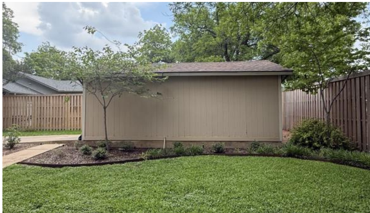
VIEW OF NORTH FACADE OF GARAGE FROM E. 10 TH STREET
