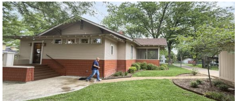
VIEW OF SOUTHWEST CORNER OF HOUSE FROM REARYARD
