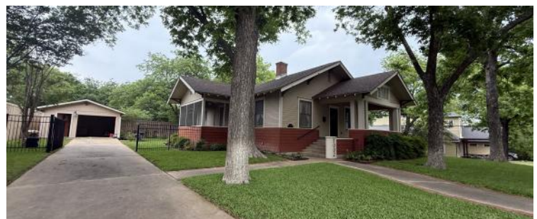
VIEW OF SOUTHEAST CORNER OF HOUSE FROM S. ELM ST.
