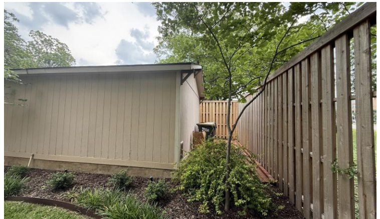
VIEW OF NORTHWEST CORNER FROM REAR YARD
