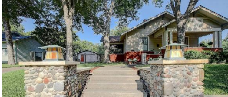
VIEW OF EAST FACADE OF HOUSE FROM S. ELM ST.
