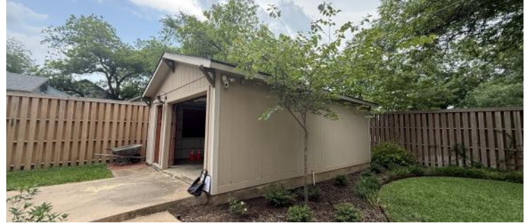
VIEW OF NORTHEAST CORNER OF GARAGE FROM SIDE YARD
