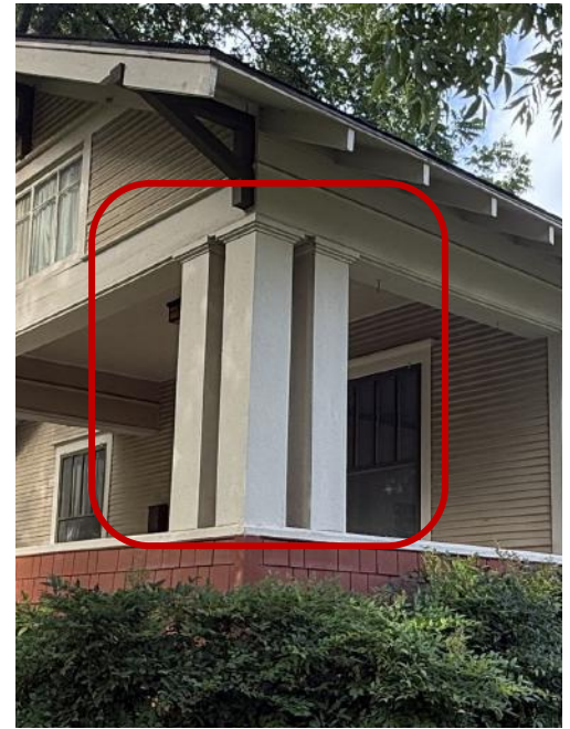
VIEW OF EXISTING CRAFTSMAN COLUMNS WITH TRIMMED TOP CAPS
