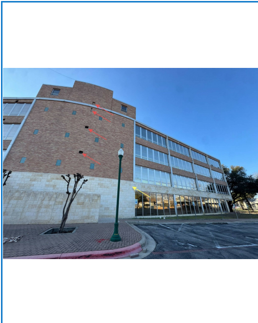
1. 02/12/2026 01:53 PM Exploratory openings in brick masonry veneer (red arrows) and limestone adhered over brick veneer (yellow arrow)
