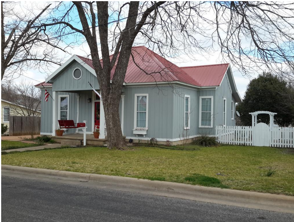
Photo direction: Northeast
