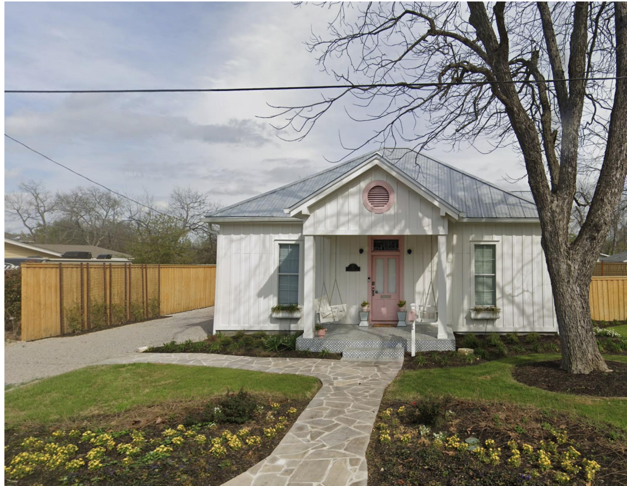
existing site photos
