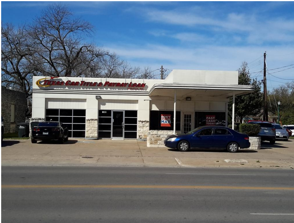
Elevation view West; Photo direction: West
