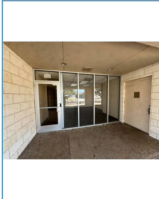
3. 02/12/2026 03:51 PM Typical aluminum, single pane, storefront style glazing
