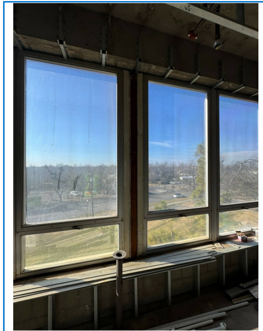
16. 02/12/2026 02:41 PM Level 4, South Elevation interior demolition around existing glazing
