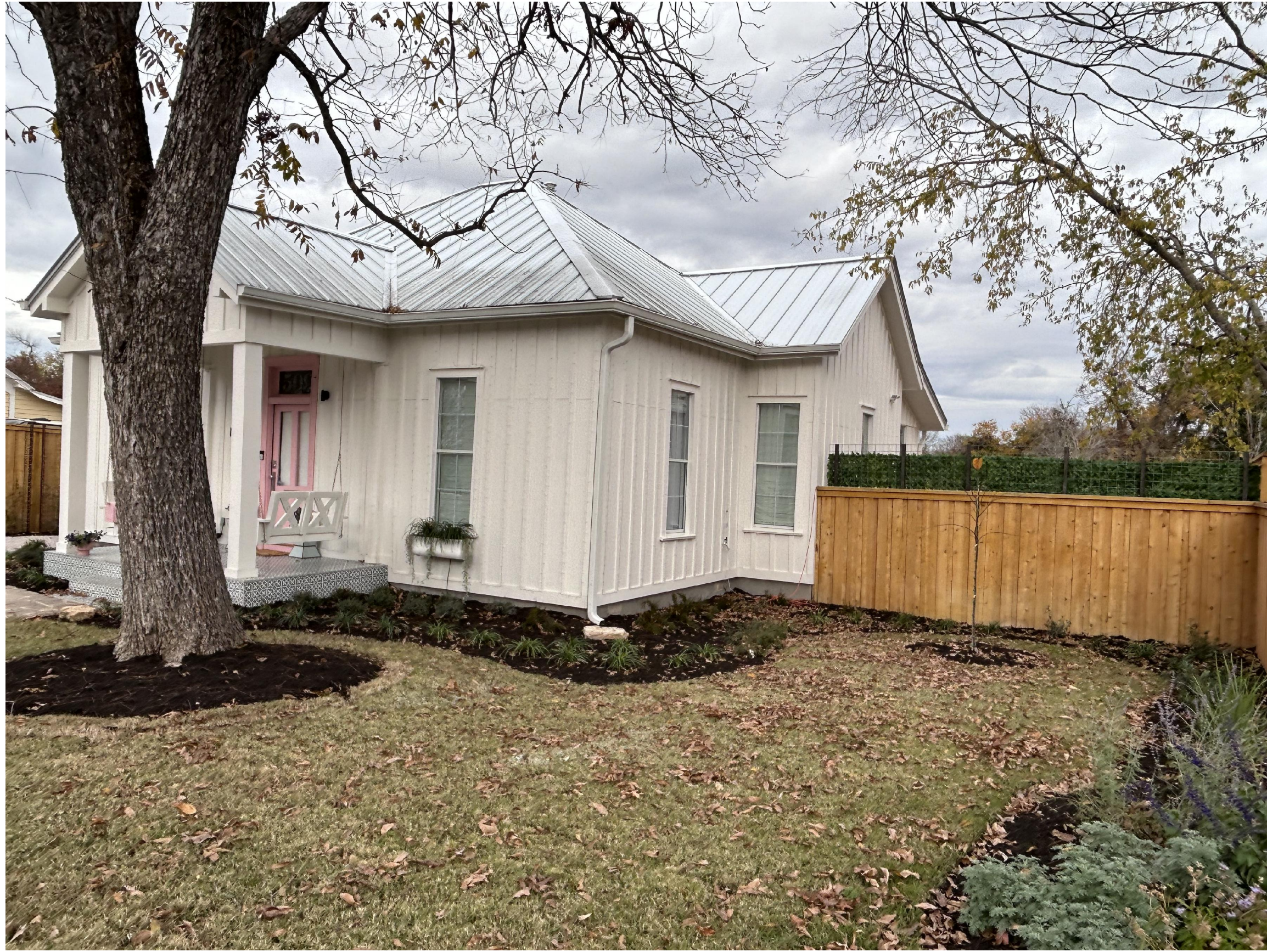
04 front-right elevation- house
