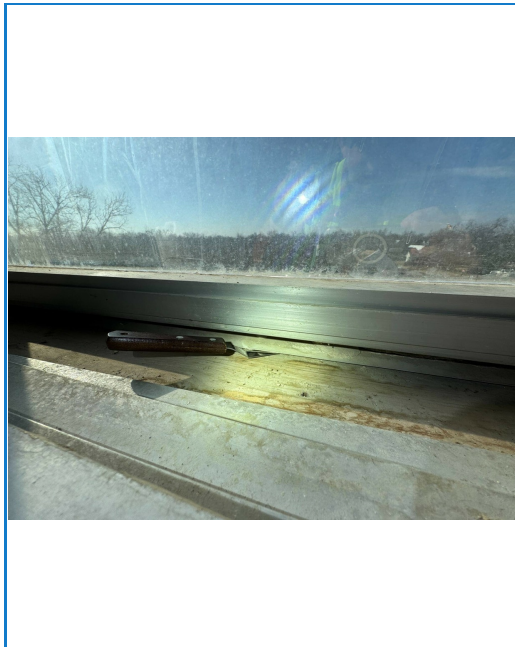
14. 02/12/2026 02:42 PM Aluminum sill extending under the glazing system, tool used to confirm no sealant is installed in the system
