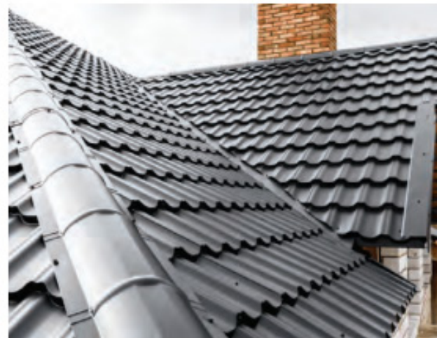
Metal tile roof.
