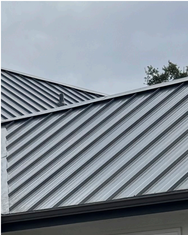
DARK METAL ROOF FROM EXISITNG HOUSE
