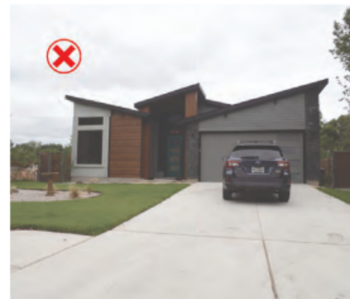
M-B: New construction incompatible with the historic district.
