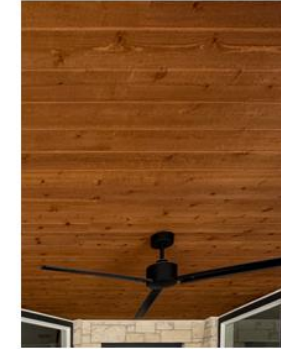
SOFFIT WOOD FROM EXISTING HOUSE
