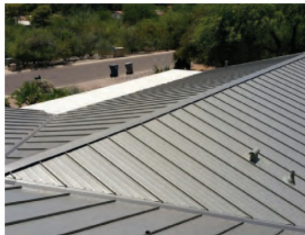
Standing seam roof.
