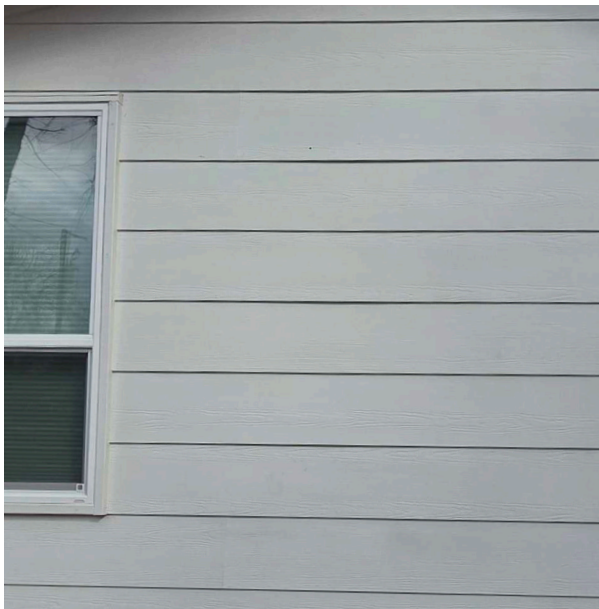
CREAM LAP SIDING FROM EXISTING HOUSE
