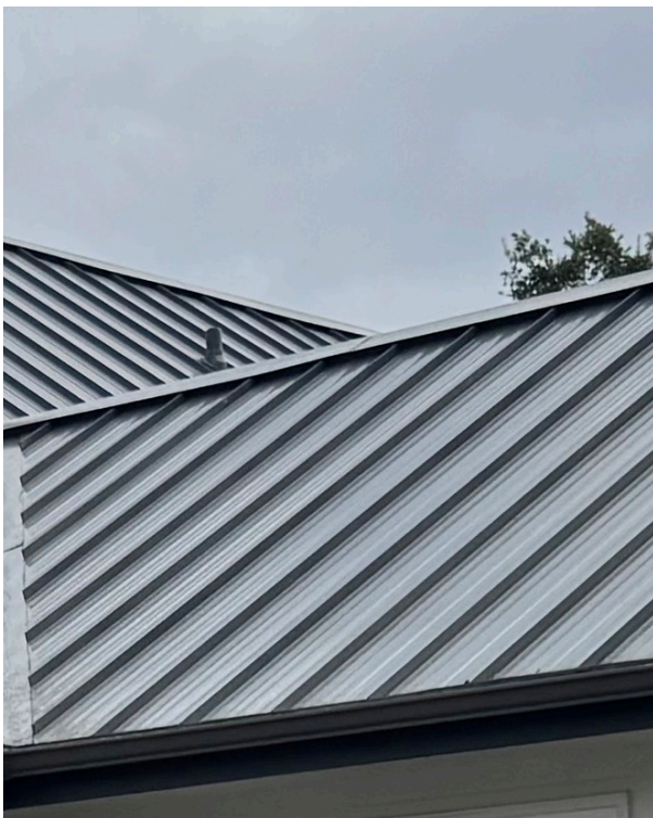
DARK METAL ROOF FROM EXISITNG HOUSE (ROOF WILL BE DOUBLE MUNCH OR DOUBLE LOCK SEAM, SPACED 18" O.C. AND NO MORE THAN 1.5" HIGH)
