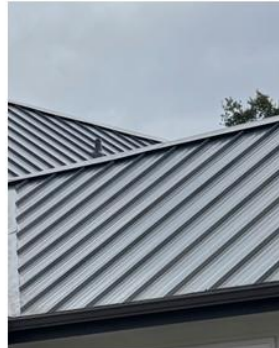
DARK METAL ROOF FROM EXISTING HOUSE
