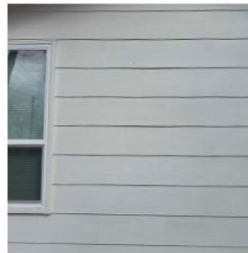
CREAM LAP SIDING FROM EXISTING HOUSE
