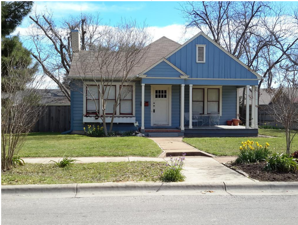
Photo direction: East
