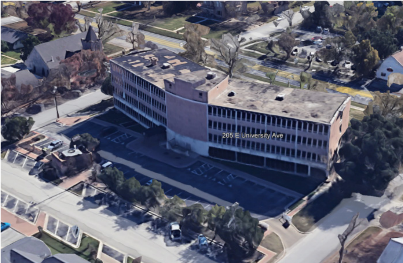
Existing Wesleyan Building
