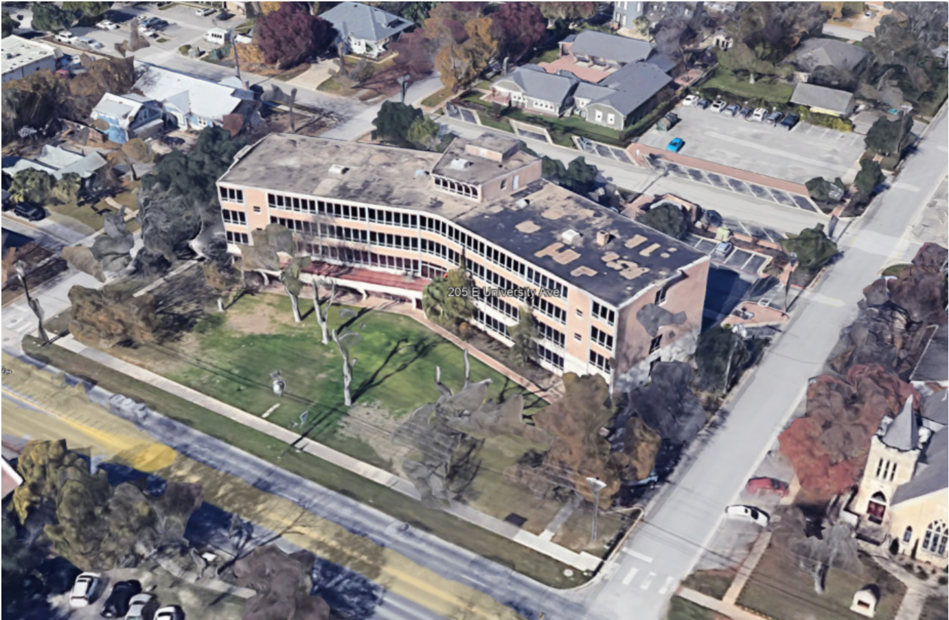
Existing Wesleyan Building
