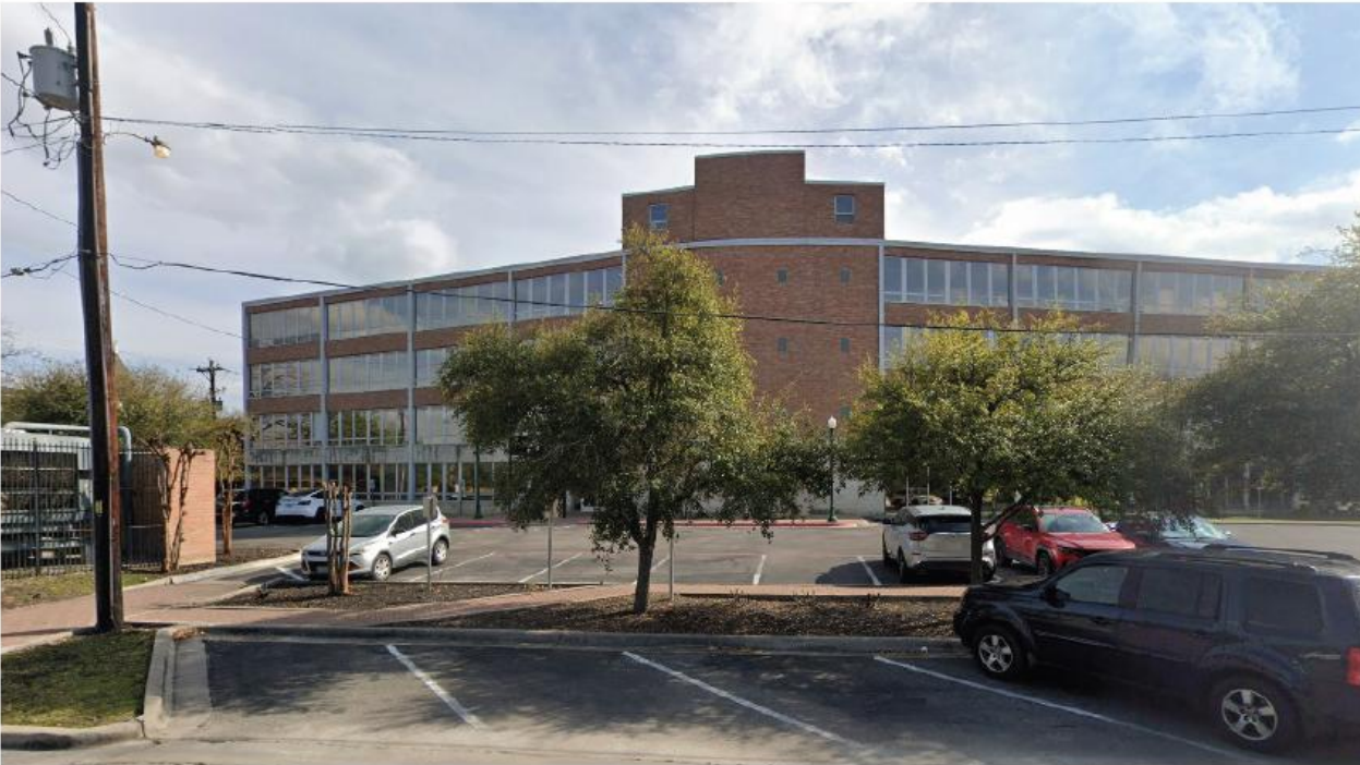
Existing Wesleyan Building
