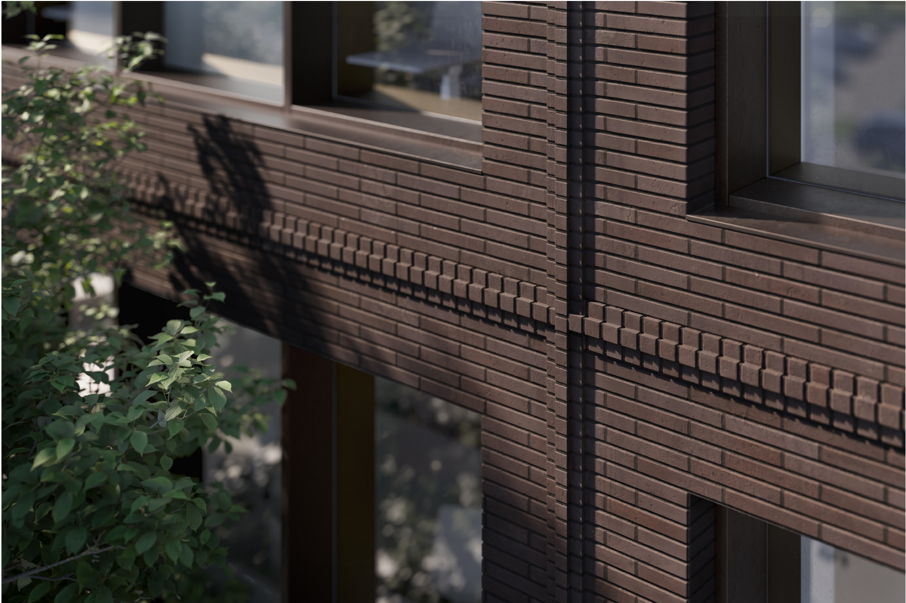
Medium Bronze Aluminum Windows @ Brick Veneer Walls
