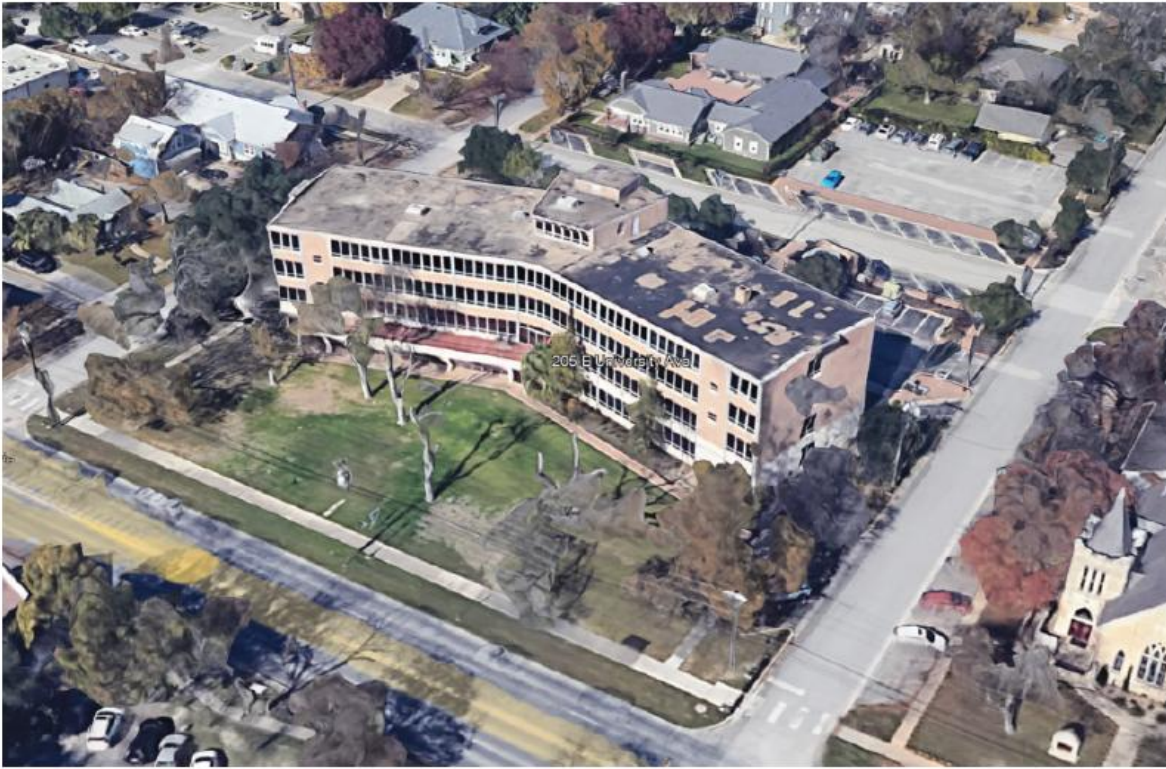
Existing Wesleyan Building
