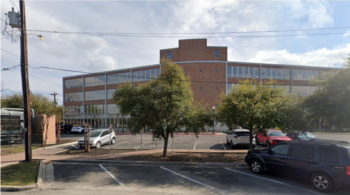
Existing Wesleyan Building
