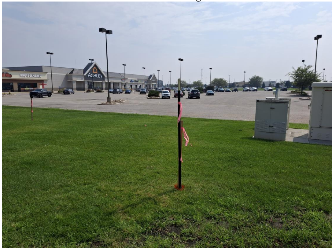
Aesthetic Pole Site looking South
