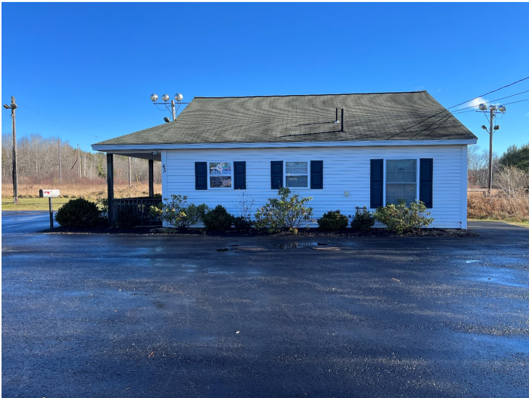
PHOTO 4 – EXISTING COMMERCIAL BUILDING
