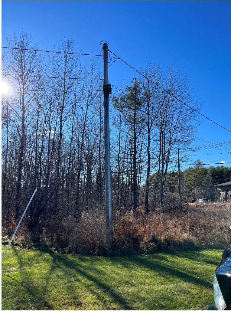
PHOTO 5 – EXISTING UTILITY POLE WITH LIGHT FIXUTER TO REMAIN.
