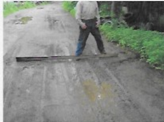
2. Driving in the same two ruts slowly pounds the road into a sort of W shape. After a rain, you can even see this effect on paved roads, especially those that are subjected to heavy trucking.
