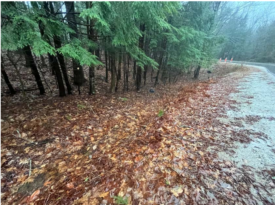
PHOTO 2 –Jenny Drive looking toward Fran Circle with existing culvert
