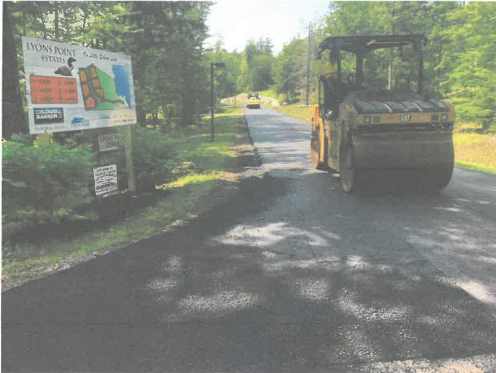
Photo #1 – Compacting 19 mm HMA with 10-ton roller, looking south
