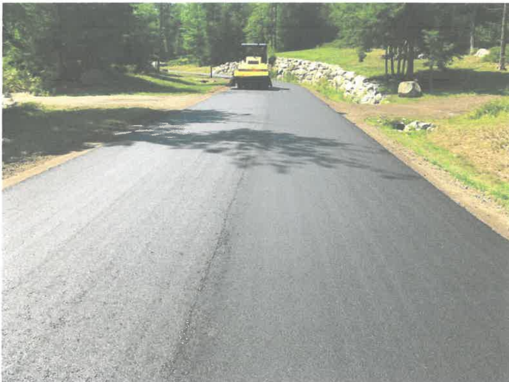
Photo #2 – Compacting 19 mm HMA with pneumatic roller, looking south
