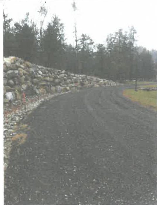
4 Road and Boulder Wall Near Lots 2 & 3
