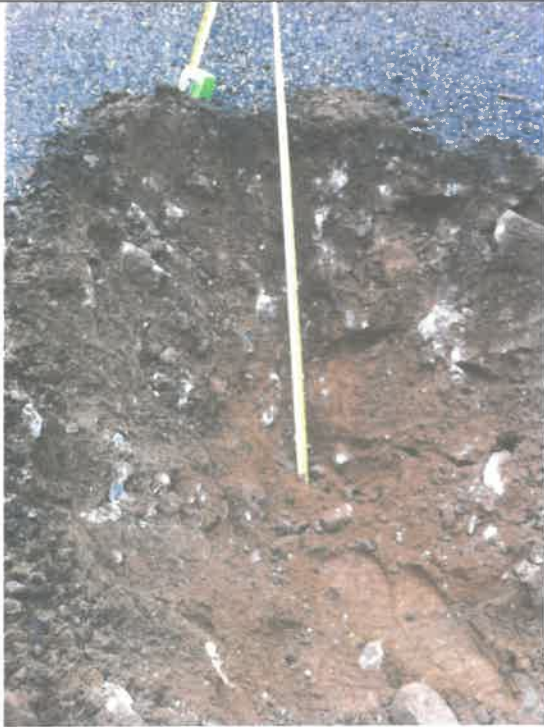
1 Test Pit #1 at Sta 1+50
