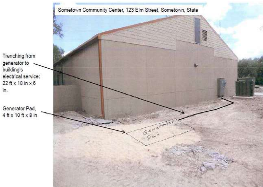
Figure 4. Ground-level photograph showing proposed ground disturbance area.
