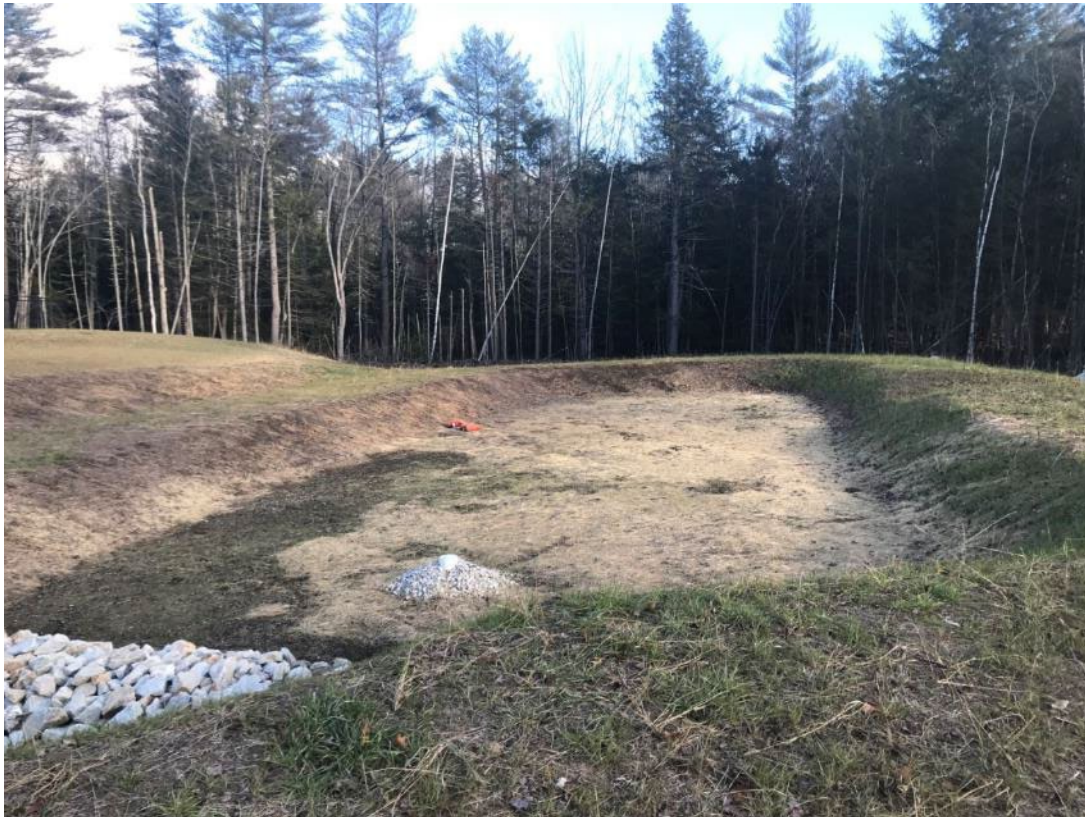
Photo 1 – View of Underdrained Soil Filter #1 (Sta. 9+50 LT, looking north)
