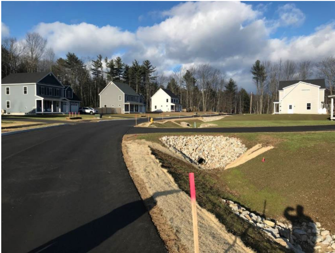
Photo 2 – View of Woodcock Drive and Ditch/Embankment (Sta. 5+50 LT, looking north)
