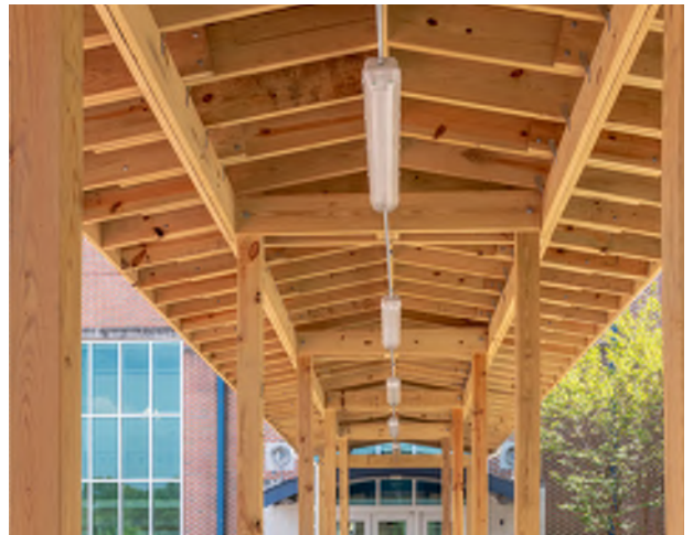
OSSE - 12115 5th Street Terminal
