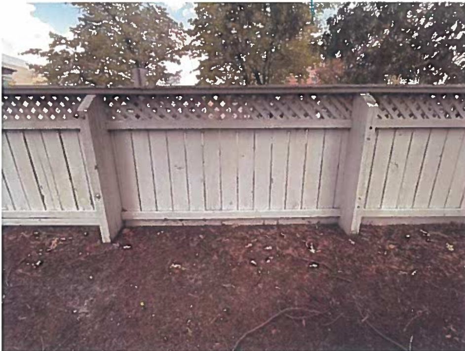
4. Existing fence on the rear side.
