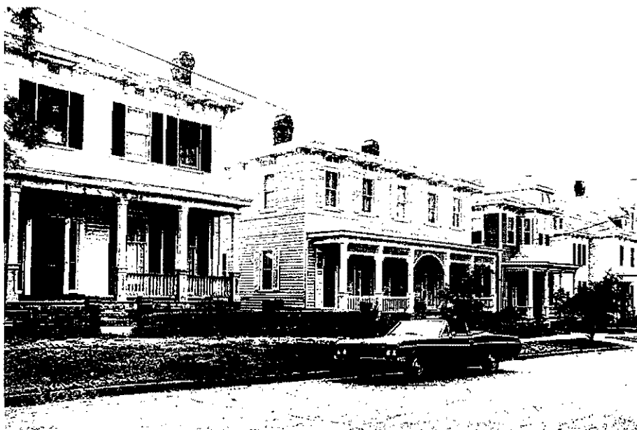
Wilmington Historic District—Residential. Established in 1962, the Wilmington Historic District Commission is one of the oldest in the state. Wilmington's six locally designated historic districts contain many excellent examples of various residential and commercial architectural styles dating from the early nineteenth century. (Shown are houses on Nun Street.)
