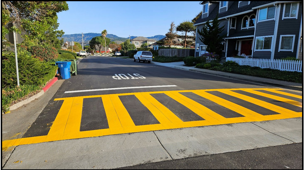
Image 2 – New High Visibility Crosswalk (facing north)
