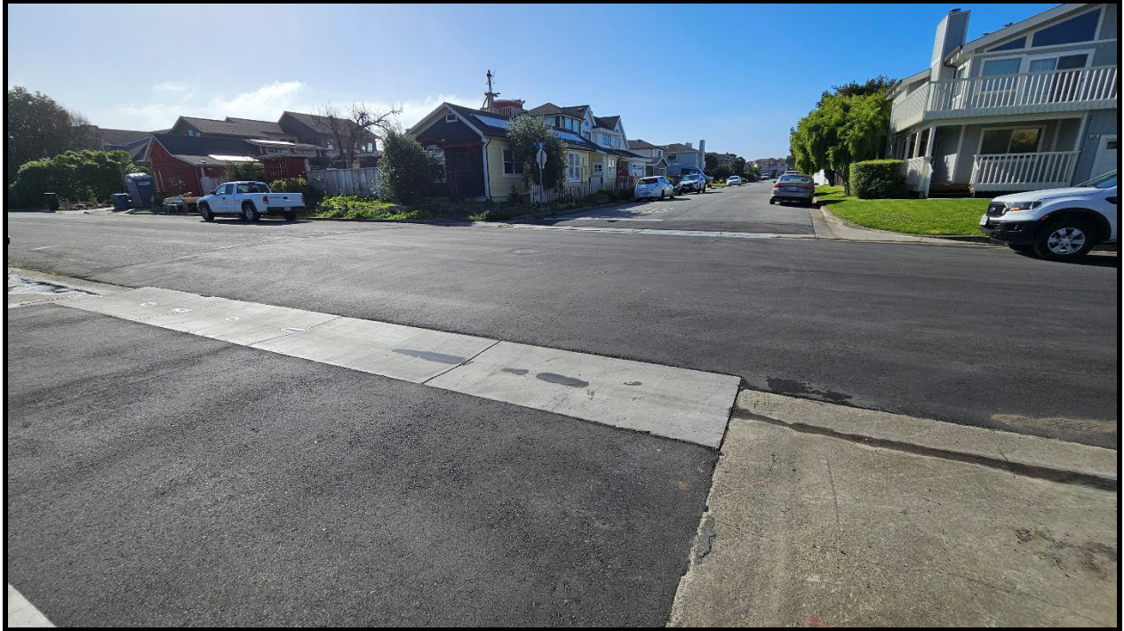
Image 4 – Potter Avenue and Valdez Avenue widened valley gutters (facing north)
