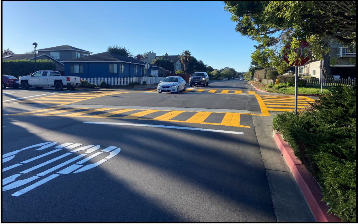
Image 1 – Alsace Lorraine Avenue Paving (facing south)
