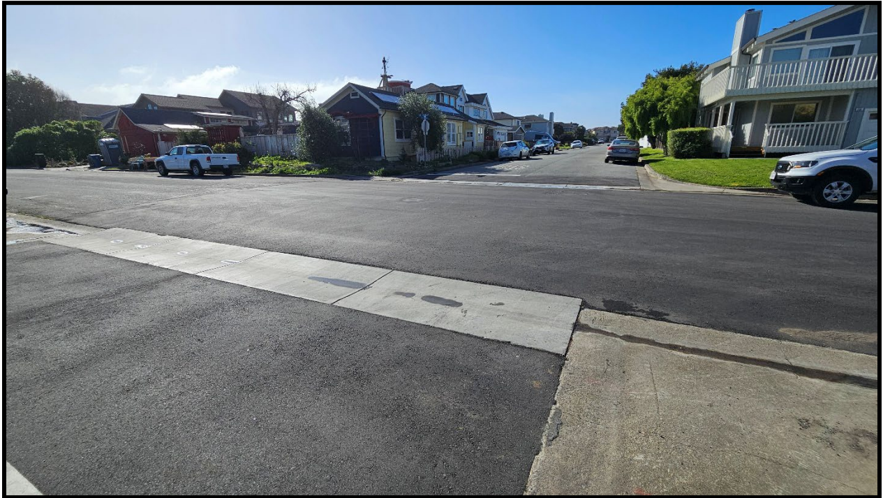
Image 4 – Potter Avenue and Valdez Avenue widened valley gutters (facing north)
