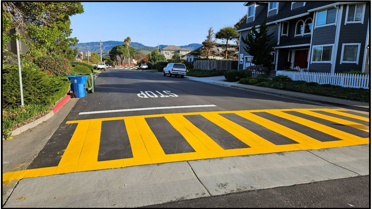
Image 2 – New High Visibility Crosswalk (facing north)
