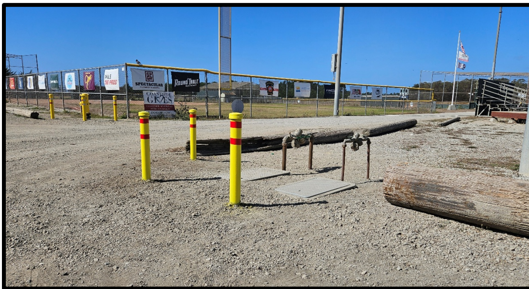
Image 3 – New Irrigation and Domestic services at Smith Field (facing north)
