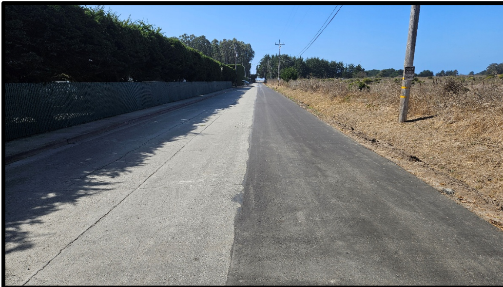
Image 1 – Wavecrest Road 10-ft trench restoration (facing west)
