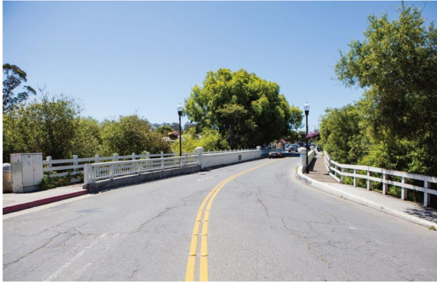
Figure 3 – Existing View of Bridge Looking South
