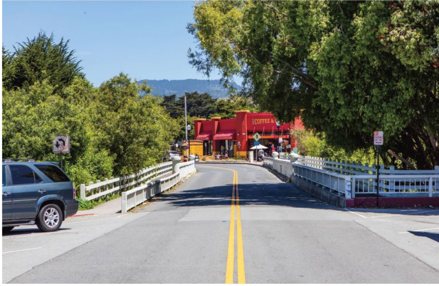
Figure 1 – Existing View of Bridge Looking North
