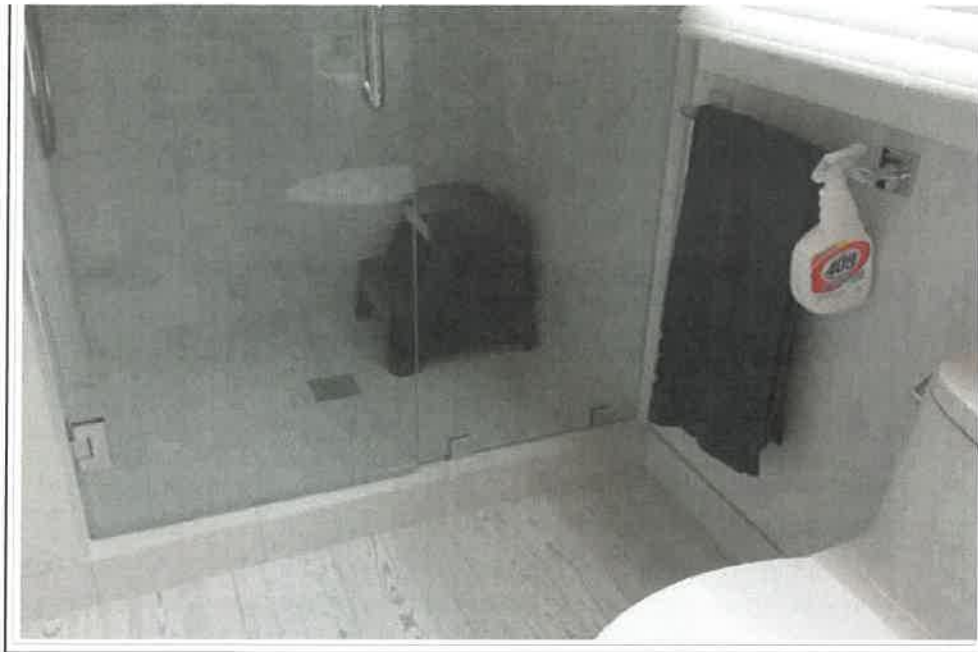
BATHROOM ADDITIONAL PHOTO
