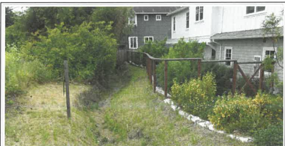
DRAINAGE CHANNEL FROM STREET
