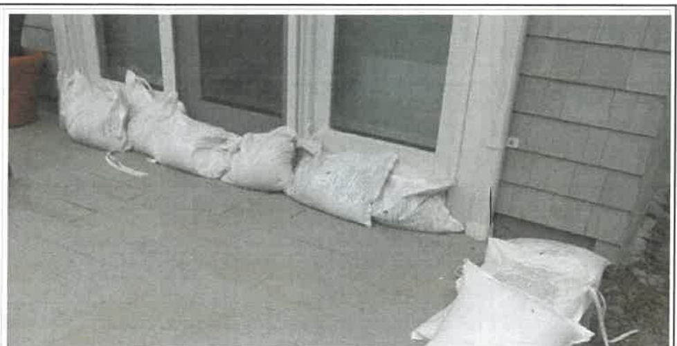
REAR SAND BAGS AT PATIO
