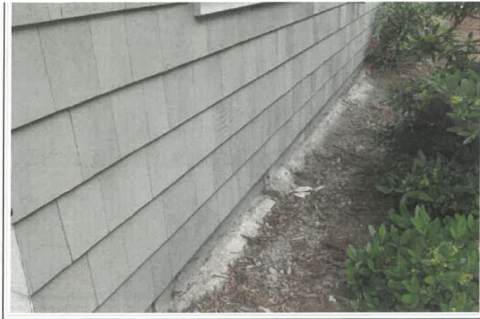
FOUNDATION AT INSPECTION ON EAST SIDE OF HOME
