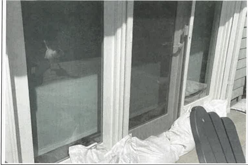
REAR SAND BAGS AT PATIO
