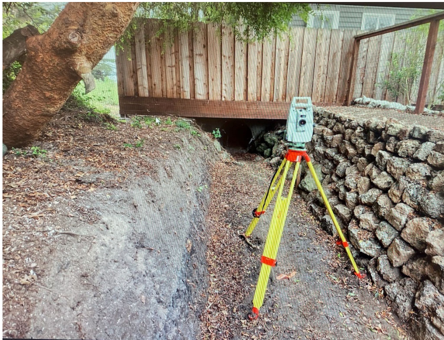
Photo #1: Looking downstream at the entrance to the culvert located on the Pullman Ditch, immediately adjacent to the proposed basin. Note that the left bank is significantly lower than the right bank in this location.
