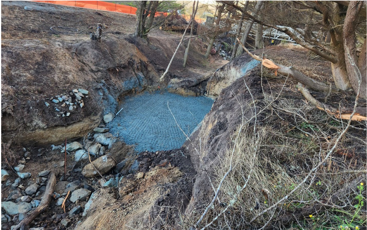
Image 2 – Compacted Base Rock at Seymour Watercourse Headcut
