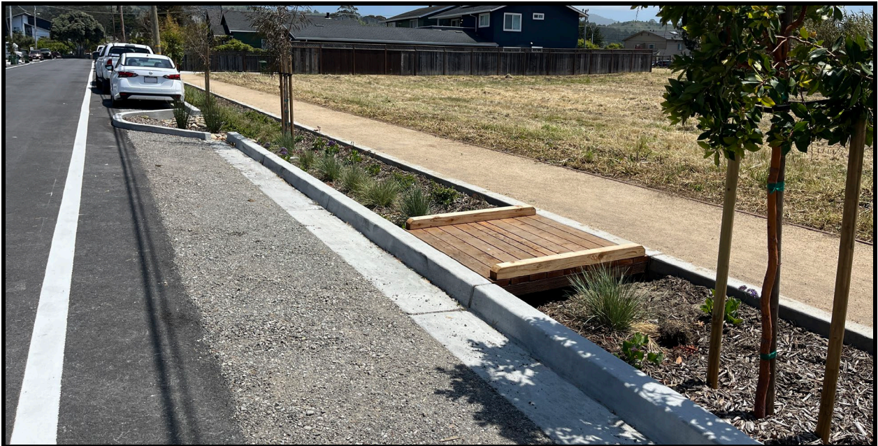
Image 2 – Pilot Platform southside (facing east)
