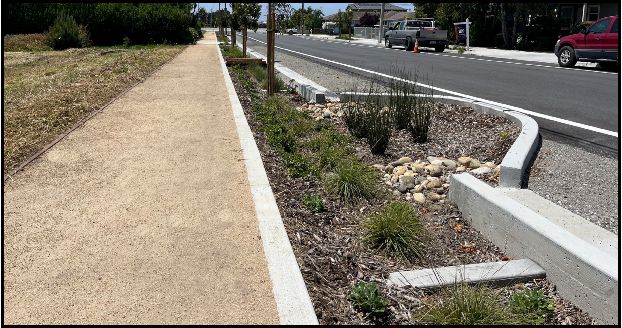
Image 1 – Bioretention Bulb-Out southside (facing west)
