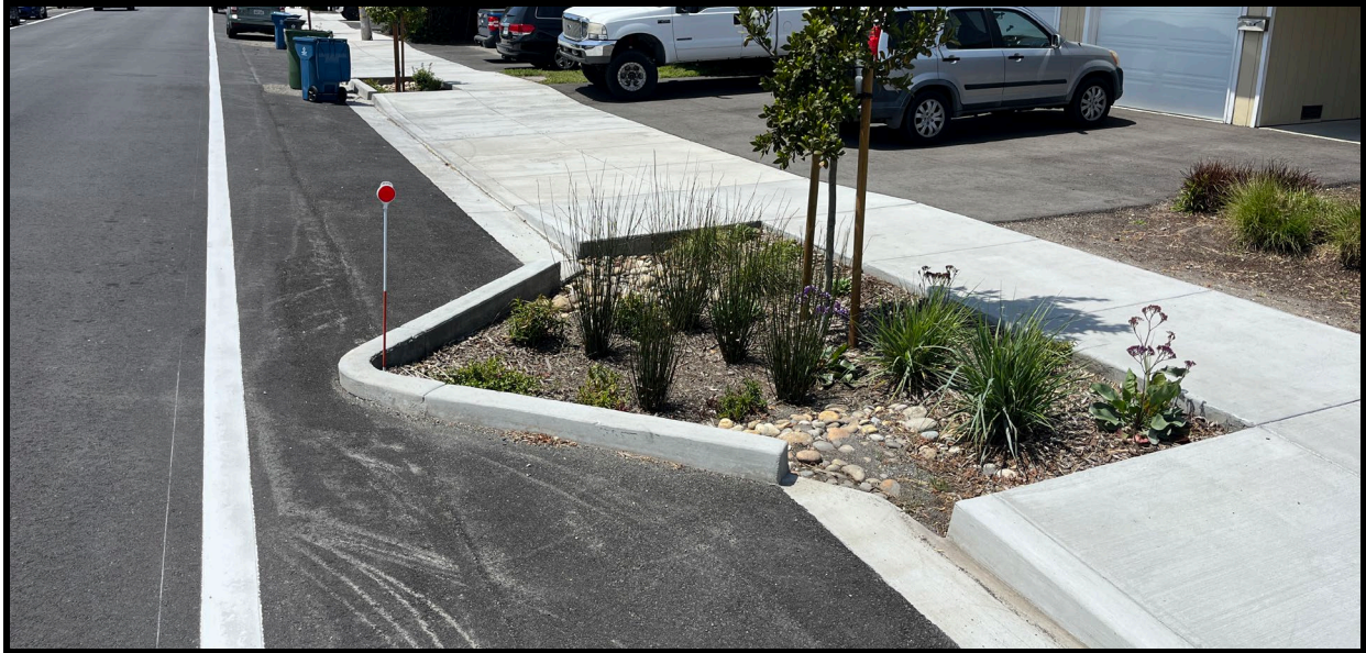
Image 3 – Bioretention Bulb-Out northside (facing west)
