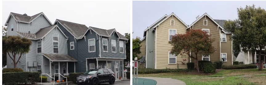
Figure 8: Main Street Park, a development built in two distinct phases. The images above show the contrasting design of the phases. The covered porches, recessed façade, and more articulation and roof and plane breaks of the older phase (left) are preferred over the simpler design approach of the newer phase (right).
