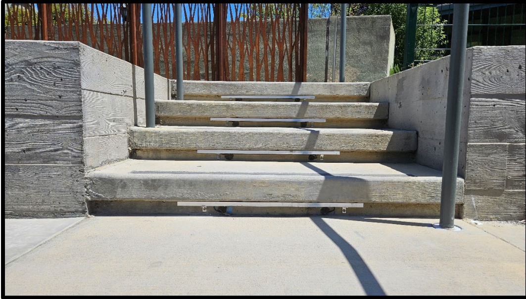
Image 3 – Amphitheater Stair Lights – Final Installation
