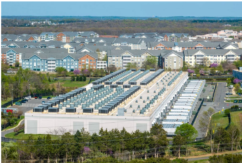
Data Center in Ashburn, VA.
