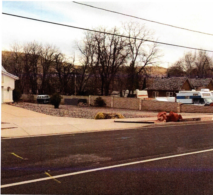
Figure 2b – Rail to Prevent Overflow of Water
