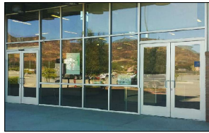
ALUMINUM STOREFRONT SYSTEM- AMF-01 – CLEAR ANODIZED ALUMINUM
