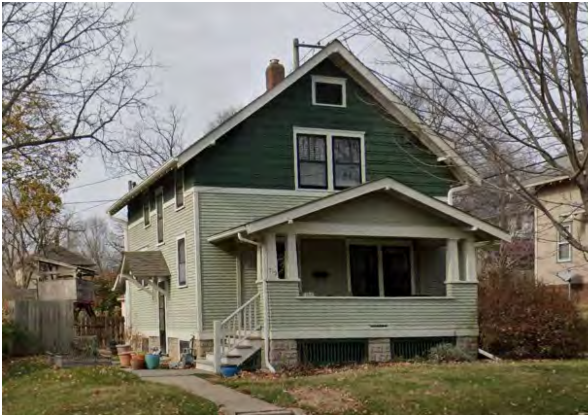
715 North Dodge Street – front façade (SE corner)
