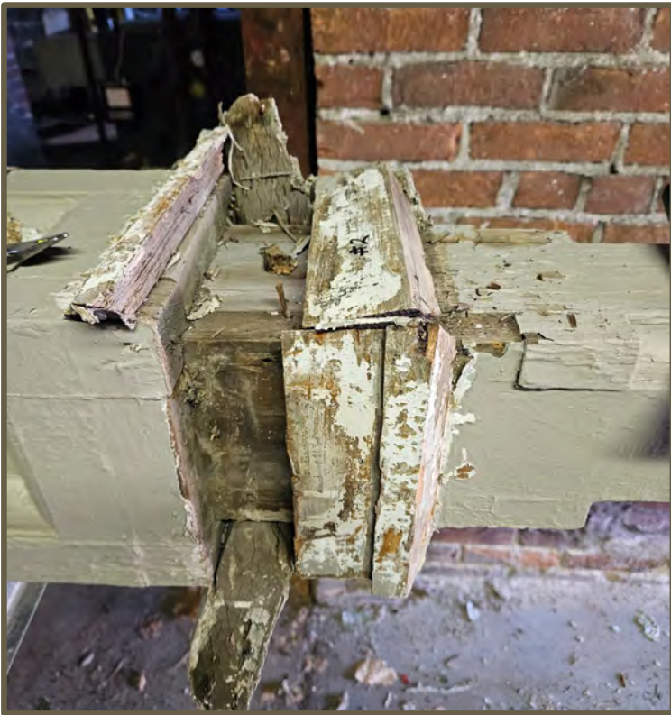
103 South Governor Street South porch reconstruction
