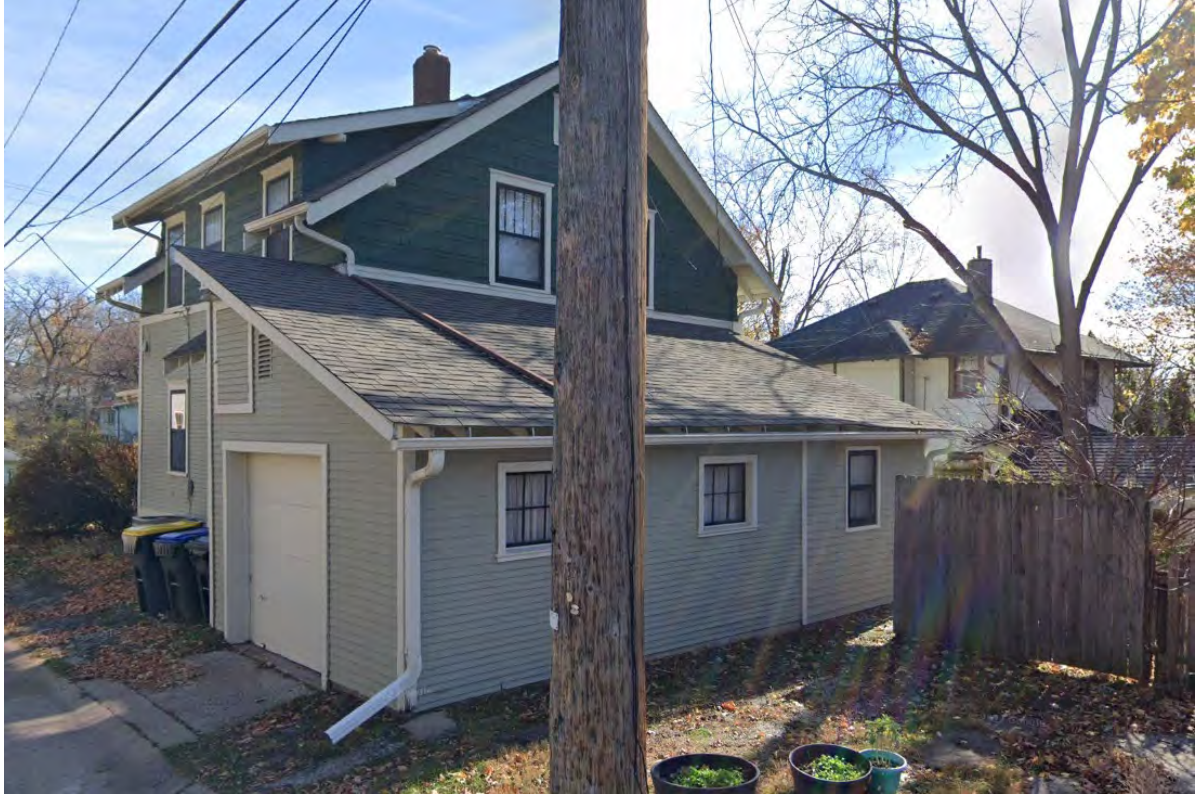
715 North Dodge Street – attached garage (NW corner)
