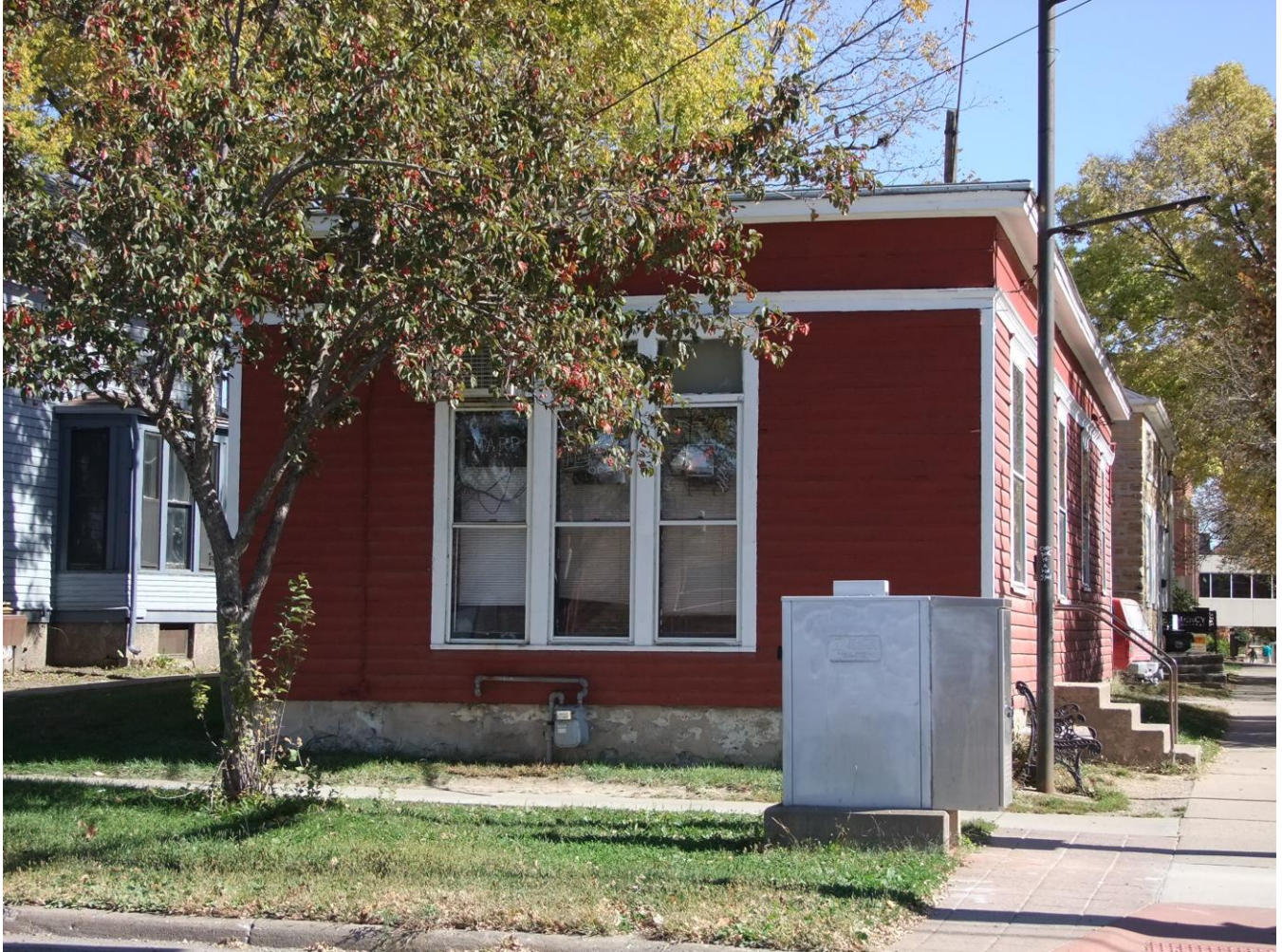
402 East Market Street – view from west
