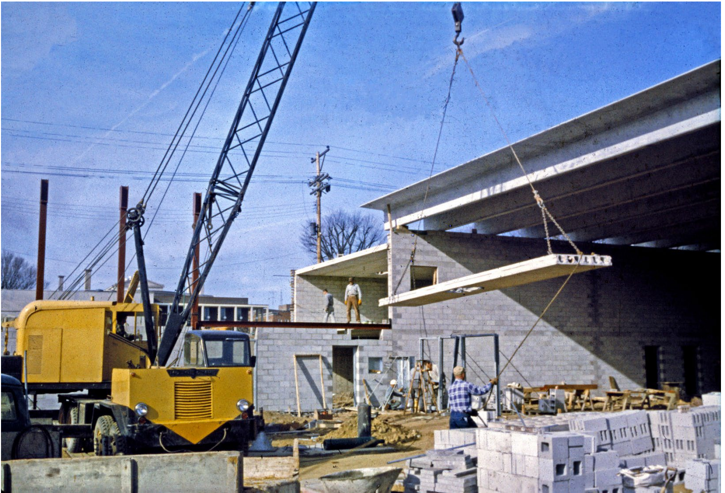
Figure 3: Placing the concrete roof panel over the north end of the gymnasium. Roland C. Wehner photo, c. 1963.
