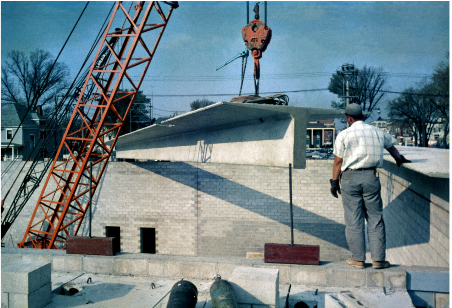
Figure 2: Placing the precast, prestressed concrete T-Beams over the gymnasium's east wall. Roland C. Wehner photo, c. 1963.
