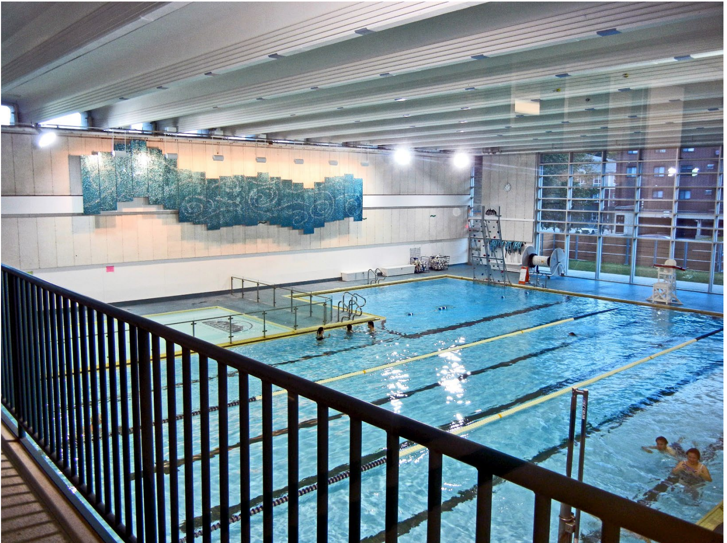
Figure 26: View from upper-level Balcony or observation deck looking east. Note the precast concrete T-beams ceiling structure. Vertical acoustical panels added to the upper walls. Glass artwork entitled "Dancing Water" glass artwork was mounted on the east natatorium wall. Roland C. Wehner photo, c. 2019.
