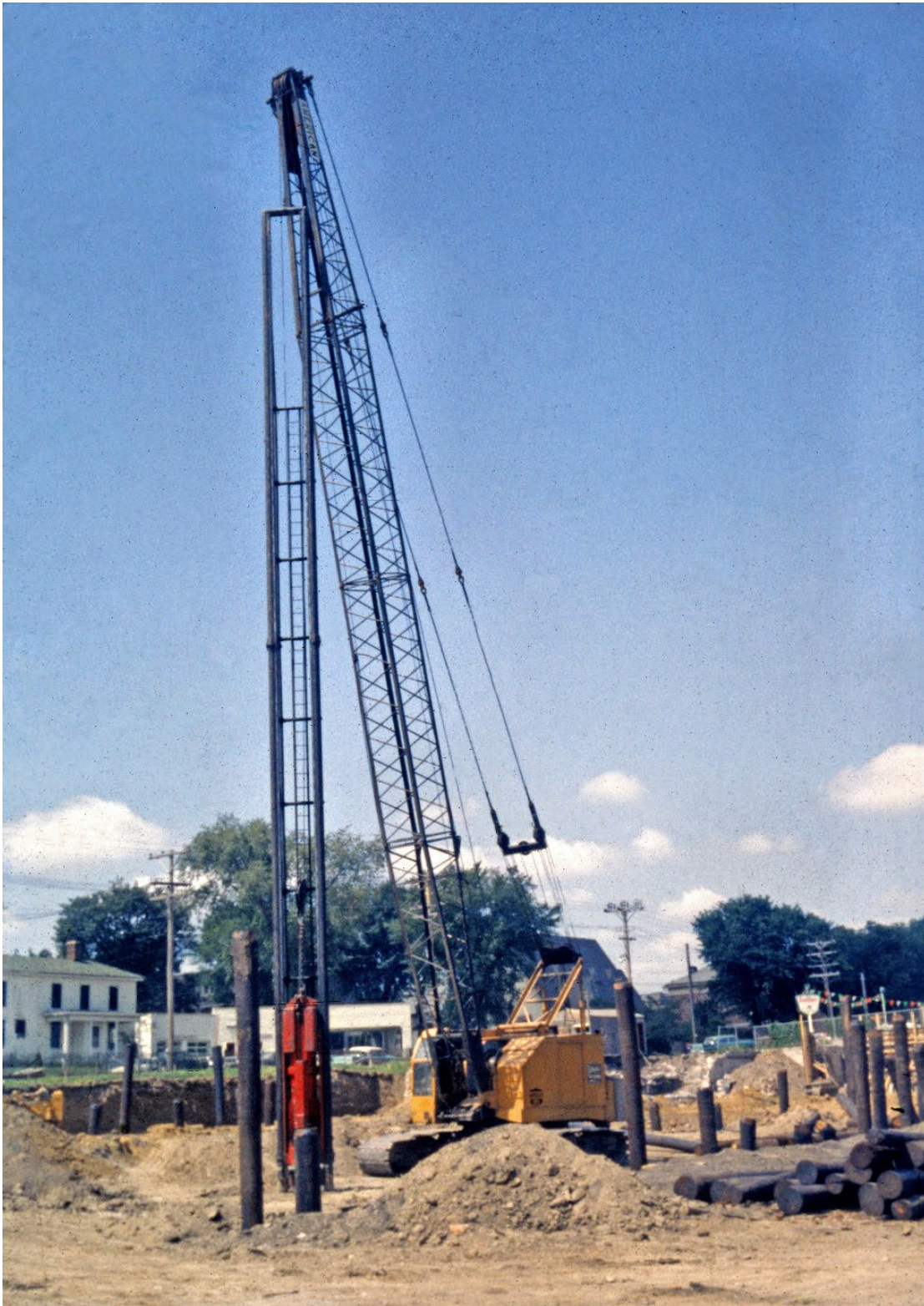
Figure 1: Driving creosote-treated wood pilings for the pool basin. Roland C. Wehner photo, c. 1963.
