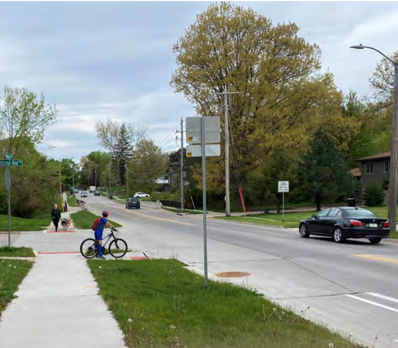
As part Iowa City’s Complete Streets Policy, bicycle lanes are considered whenever arterial streets are reconstructed or extended. The image above shows new bike lanes on Rochester Avenue.
