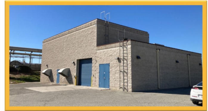
Fig 3.2: Aeration Blower Building
