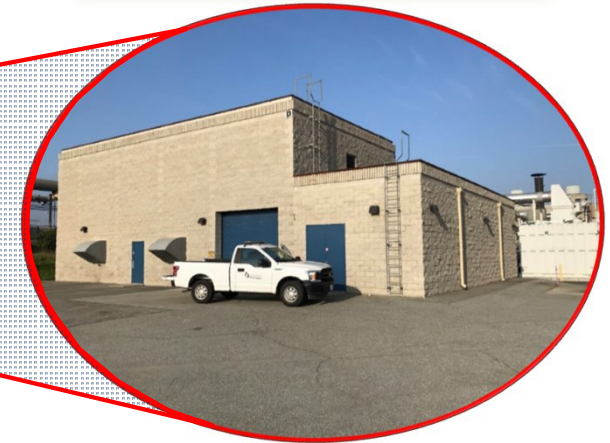
Aeration Blower Building
