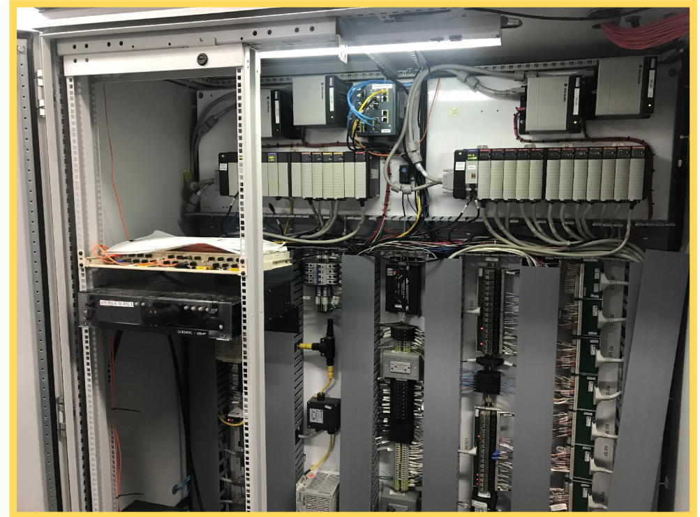
Programmable Logic Controllers
