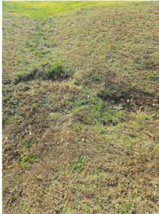
Stable erosion at inlet swale to Basin 2.
