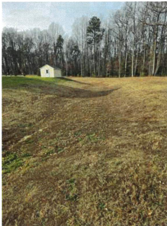
Infiltration Basin 2 looking north.
