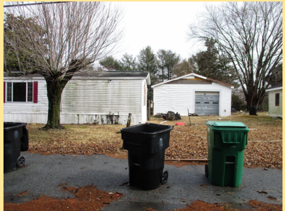
A-26-06 BIGG JIM'S HOMES LLC
