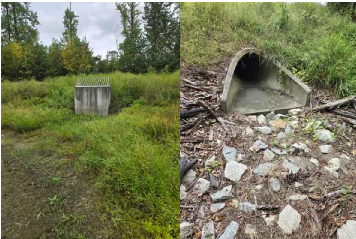
Pond 4 outlet structure.
