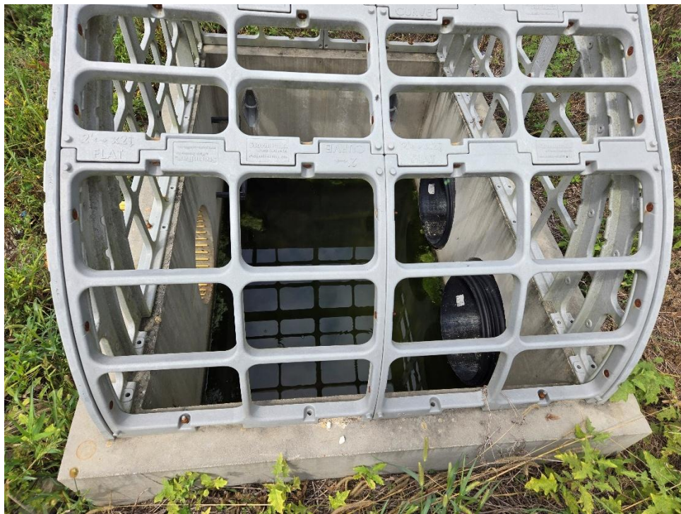
Pond 1 outlet structure holding water.
