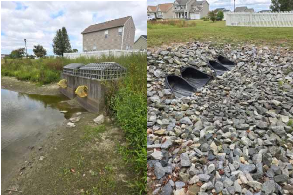
Pond 5 Outlet structures.
