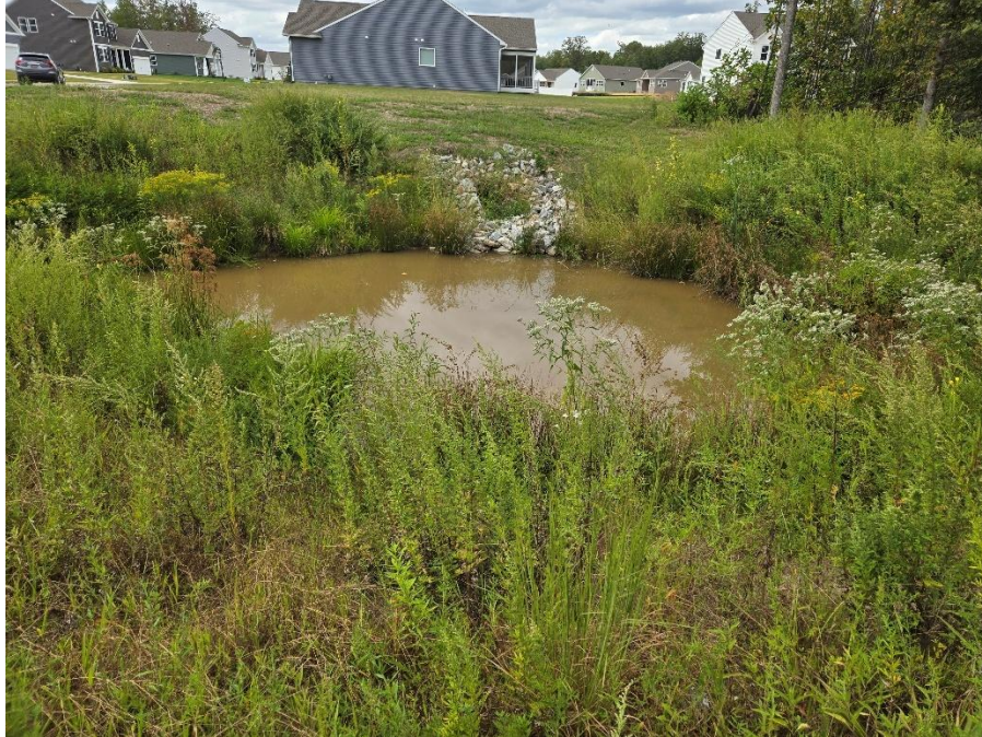
Pond 3 inlet with vegetation to be cut.
