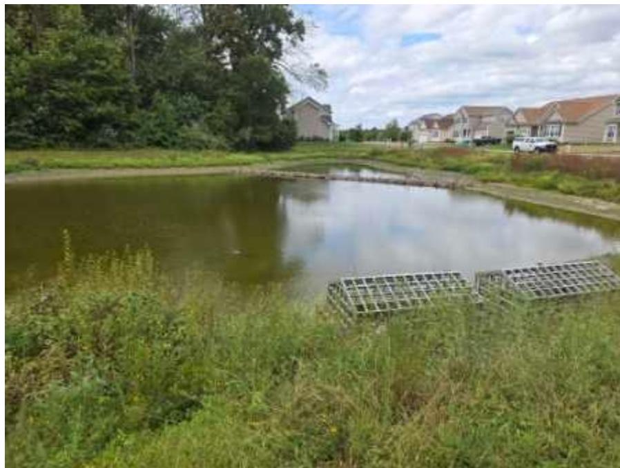
Pond 5 looking towards inlets.
