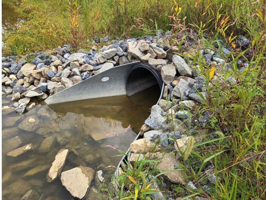
Pond 3 inlet with metal flared end section.
