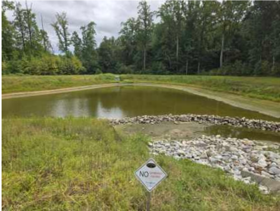
Pond 4 looking towards outlet structure.
