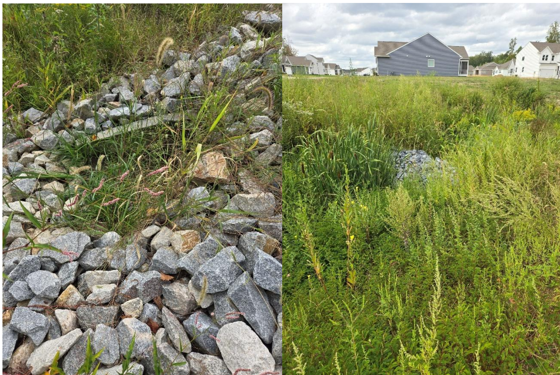
Pond 3 inlet into swale and check dam.
