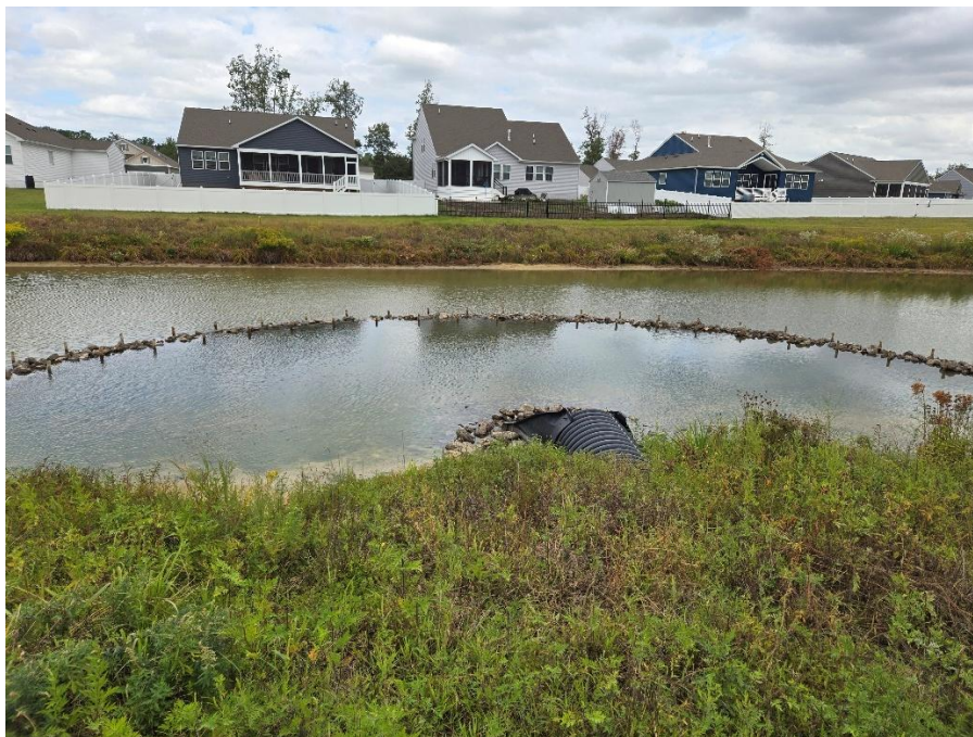
Pond 2 inlet and gabion forebay.
