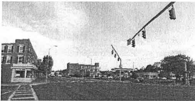
Figure 2: Traffic and pedestrian signals will be upgraded and improved.
