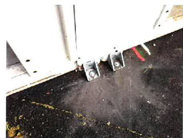
2 tie downs per corner (maybe one per corner is enough?)
