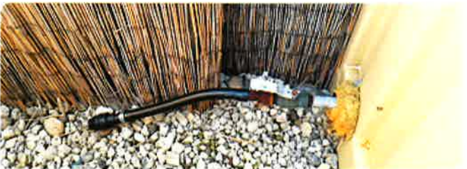
WATER HOOK UP
