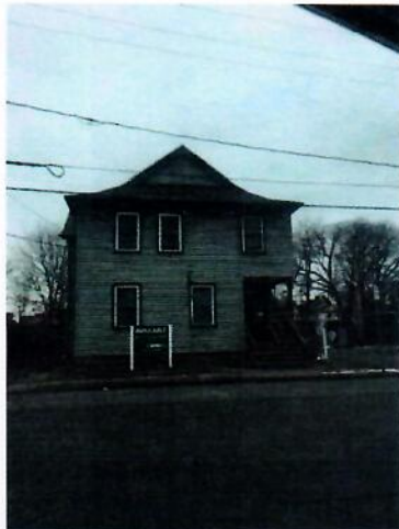
Photo A Front of Building Taken 1/31/20 1:50pm
