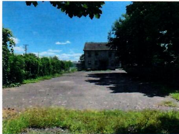
Photo B View of Rear Yard and Rear of Building Taken 8/20/20 1:12pm
