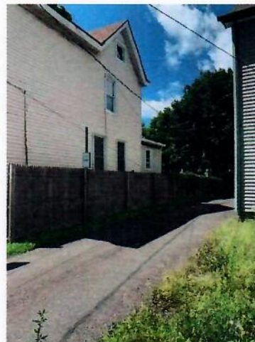
Photo D Side View of Driveway Taken 8/20/20 1:13pm
